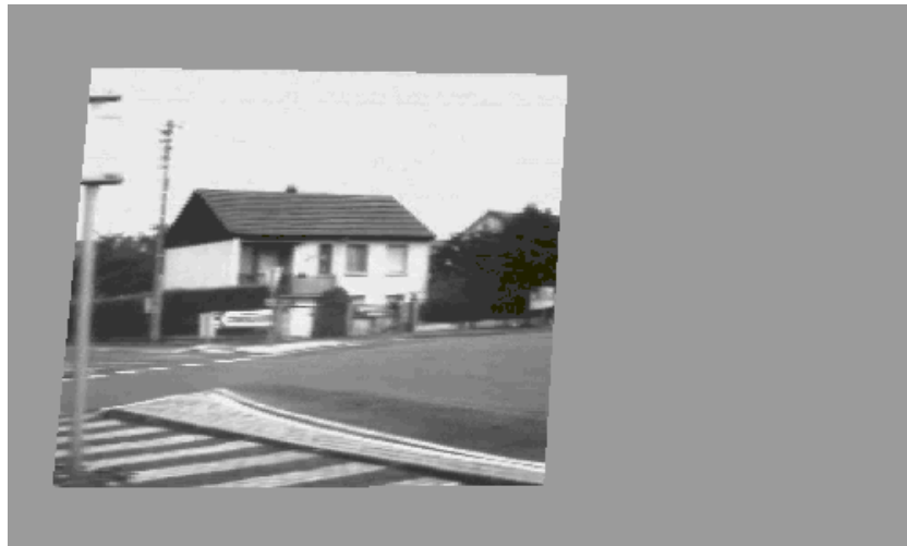
The house façade is stabilized
